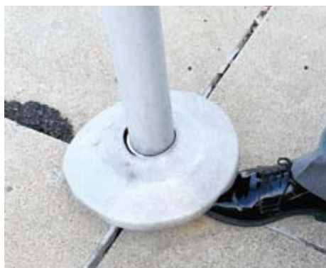
The cement under the American flag pole has sunk so far a shoe can fit underneath.
