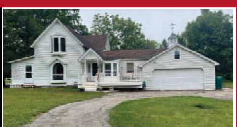
13300 EDGEDALE, VAN BUREN TOWNSHIP
