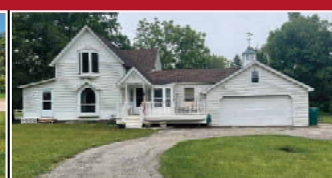
13300 EDGEDALE, VAN BUREN TOWNSHIP
