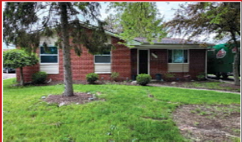
1112 JACKSON VAN, BUREN TOWNSHIP 1163 SQUARE FOOT BRICK RANCH with 3 bedrooms plus dining area. Many Updates include Central Air, Vinyl Windows, Flooring, Deck, Gutters and Driveway. 209,000
