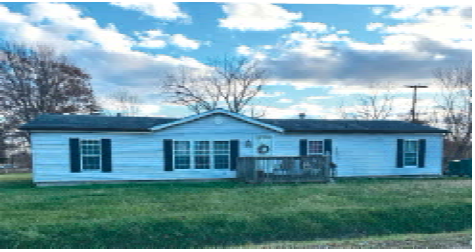
29515 CHARLES, ROMULUS IT'S LOADED WITH 4 BEDROOMS, 2 Baths, 1,647 Square Feet, Fireplace, Deck and More. On 1/2 Acre with Huge Garage. 1996 Construction Just $200,000
