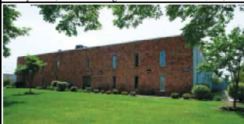
12950 HAGGERTY VAN BUREN TOWNSHIP FOR LEASE Zoned M-2 for many uses. Best location with 16,800 Sq Ft For Lease. 20 Foot Ceilings, Large Offices Huge Work Area. Close to I-94 & I-275. $6,900. Mo Triple Net
