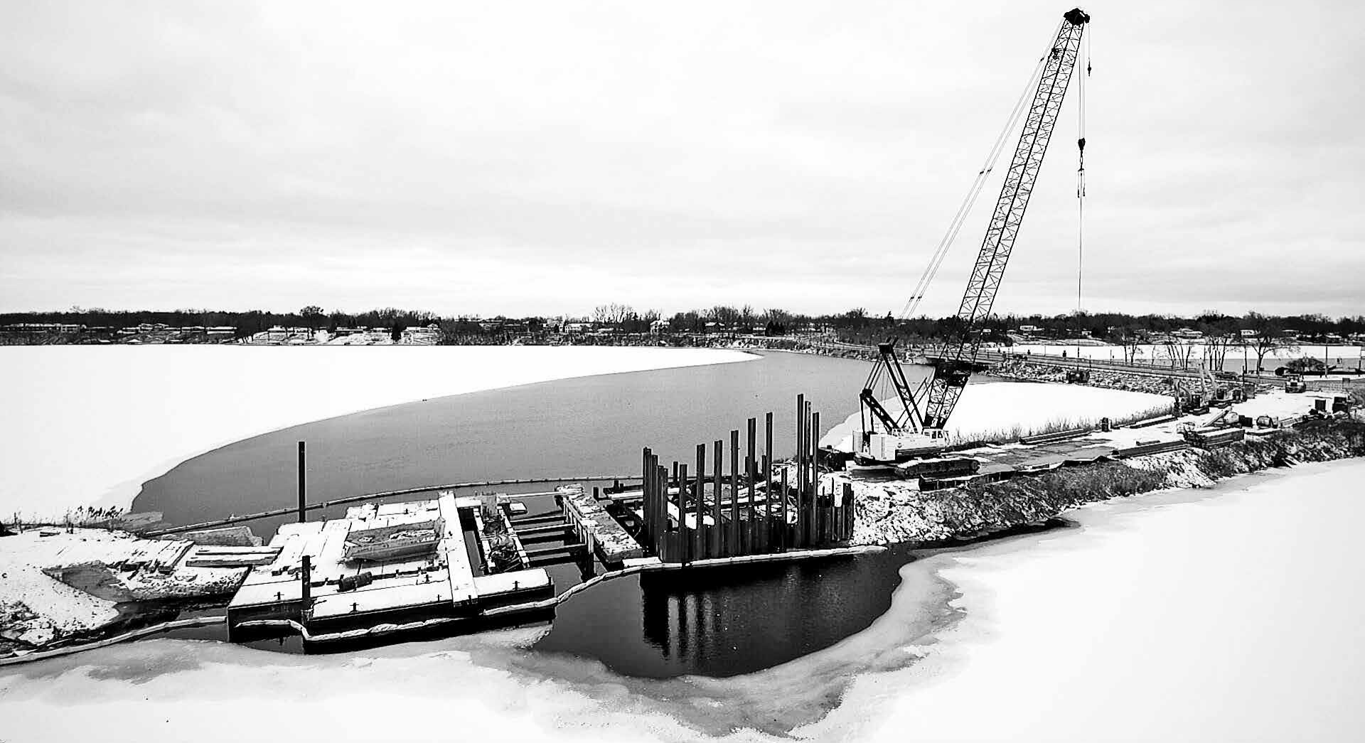
Work progresses on the Denton Road Bridge even in the icy weather over the weekend.
