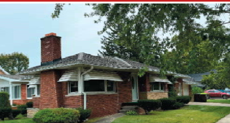
208 E HURON RIVER DR, BELLEVILLE CITY OF BELLEVILLE BRICK RANCH with 3 Bedrooms, 1 1/2 Baths, Fireplace, Dining Area, Large Living Room, Full Basement 1,385 Sq Ft Attached Garage $215,000
