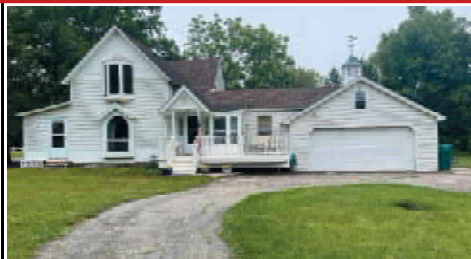
13300 EDGEDALE, VAN BUREN TOWNSHIP
